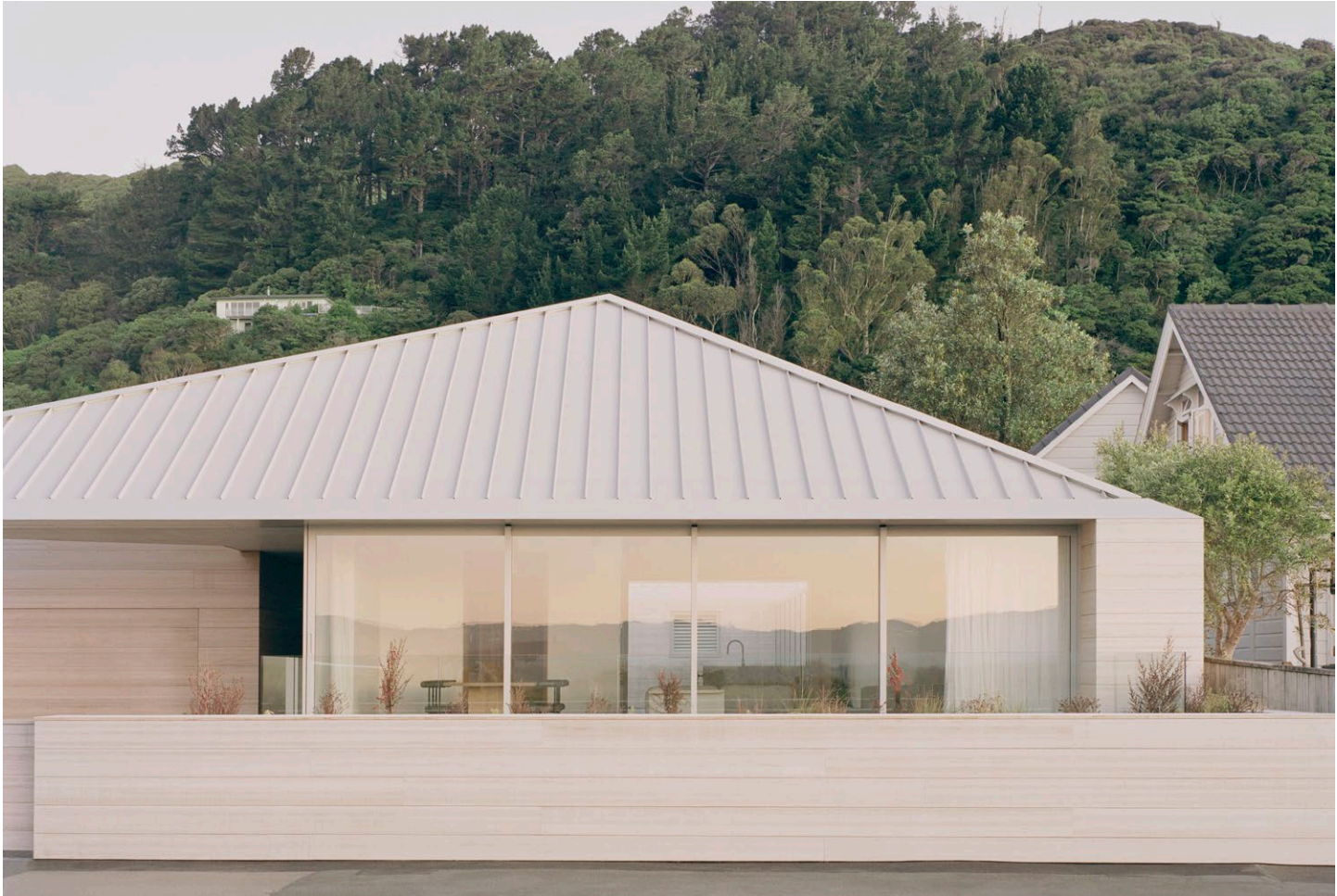
New Zealand pine cladding, selected for its likeness to driftwood, expresses a rough-textured finish and greyish hue attuned with the environment.
